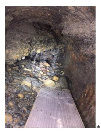
In the photo above you can see the rock debris in the bottom of the pipe plus there is a large mass of concrete in the top half that is thought to be the cause of all the debris getting trapped in the pipe. It is not known how the concrete made its way into the pipe but it is suspected that during patio construction above it may have leaked in through an opening somehow when footings were being poured.
