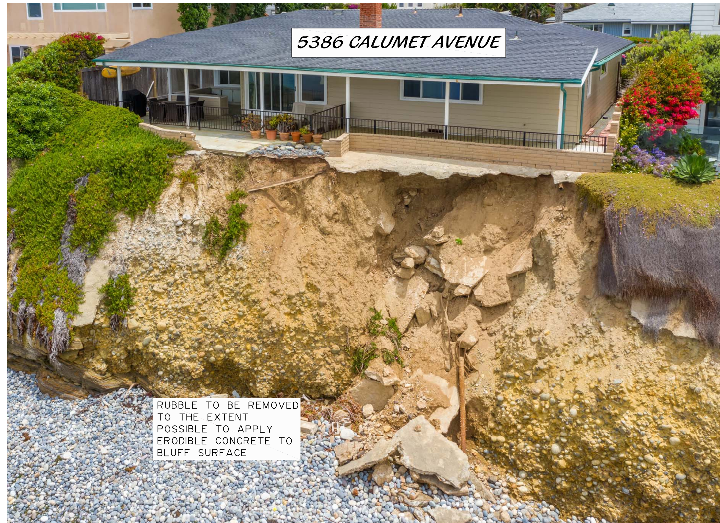
DRONE PHOTO - EXISTING CONDITION
