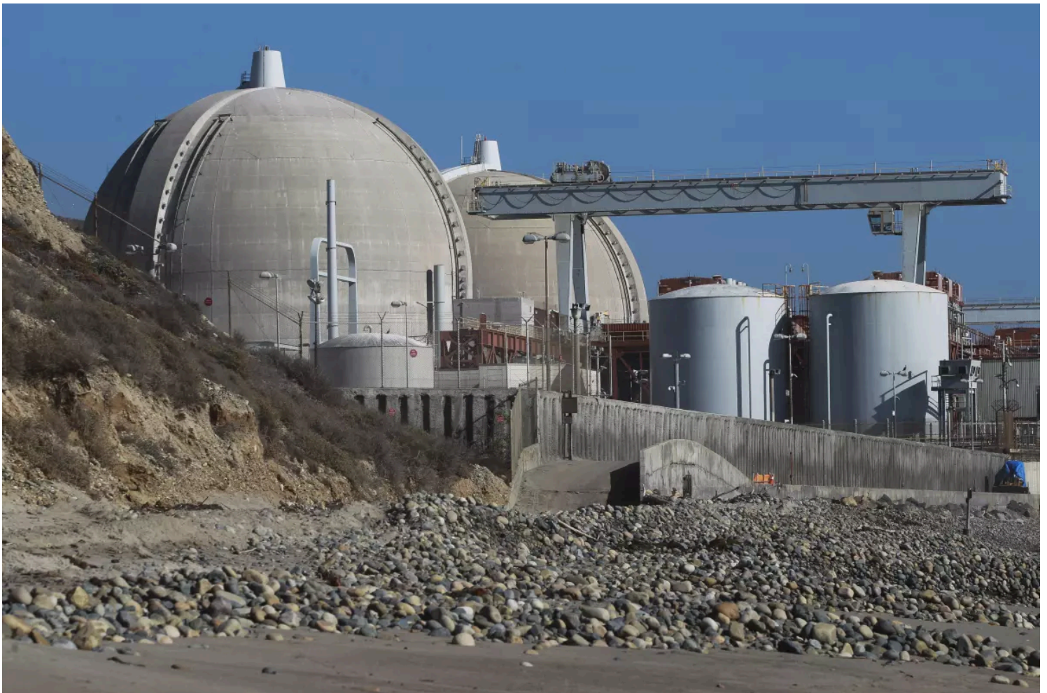
The San Onofre Nuclear Generating Station viewed from San Onofre State Beach, California on Thursday, October 17, 2019. (Hayne Palmour IV/The San Diego Union-Tribune)
