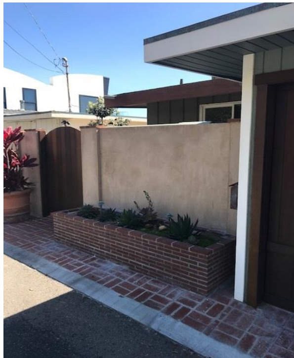
wall at house
