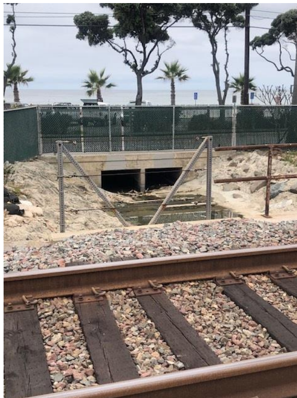
seaward view where the drain goes under the road
